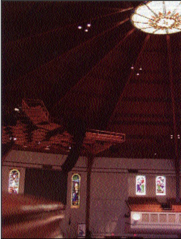
***A central line array hangs close to the center of the dome to control sound to the main floor seating area.***
